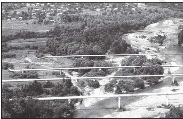
Fig. 7.17: Pipelines transporting natural gas in Ukraine
