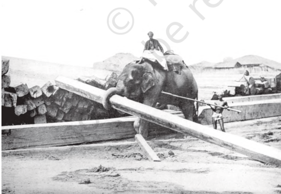
Fig.5 – Elephants piling squares of timber at a timber yard in Rangoon. In the colonial period elephants were frequently used to lift heavy timber both in the forests and at the timber yards.
