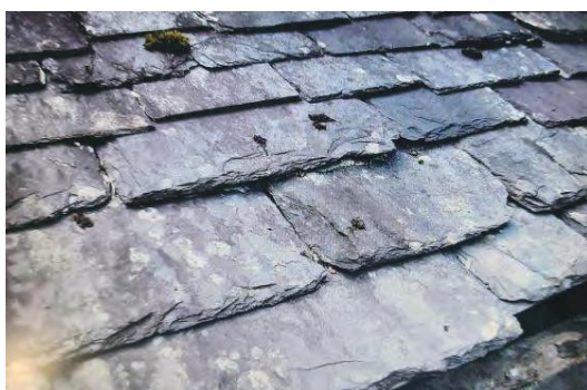
Fig. 11.6: Rocks used for roofing
