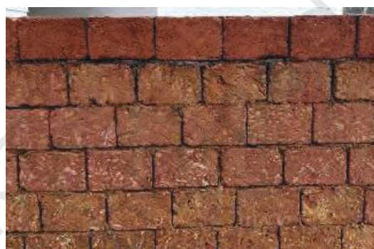
Fig. 11.7: Laterite rocks used as bricks
