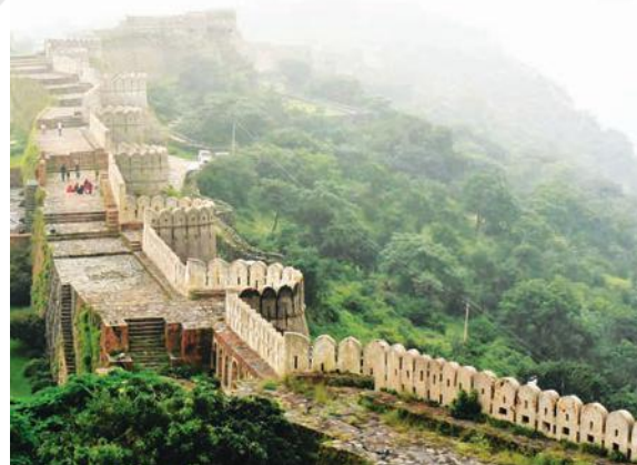
Fig. 1.26. Kumbhalgarh Fort surrounded by the Aravallis; this location in the hills proved to be an excellent deterrent to the enemy.
