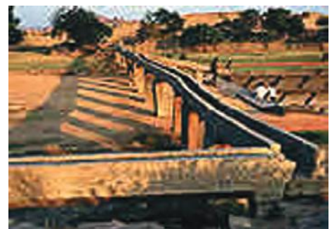
Fig. 7.5 An aqueduct leading into the royal centre
