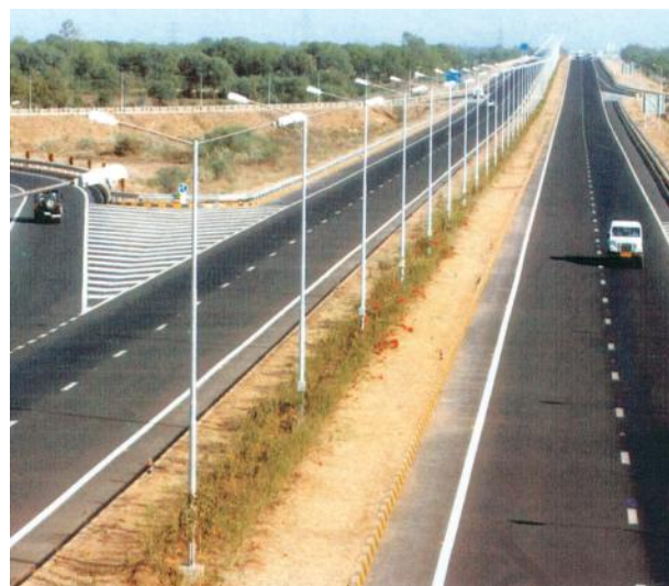
Fig.7.2: Ahmedabad- Vadodara Expressway
