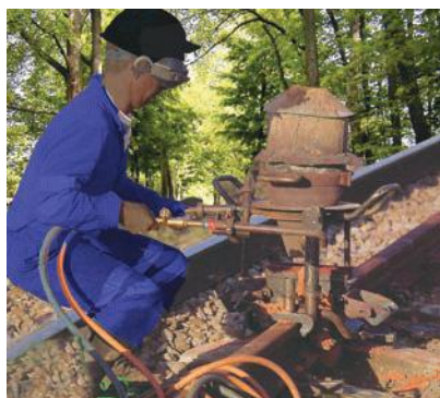
Figure 3.11 Thermit process for joining railway tracks
